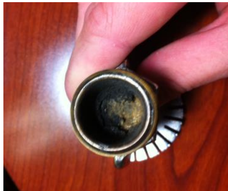
Failed Sprinkler Head (Illinois, 12 year old system )
