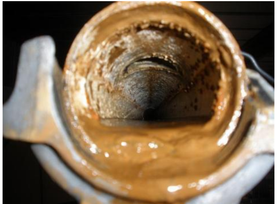
Typical “Dry” System
