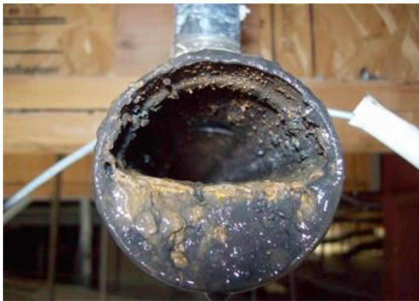
50% Blockage (California, 5 year old system )
