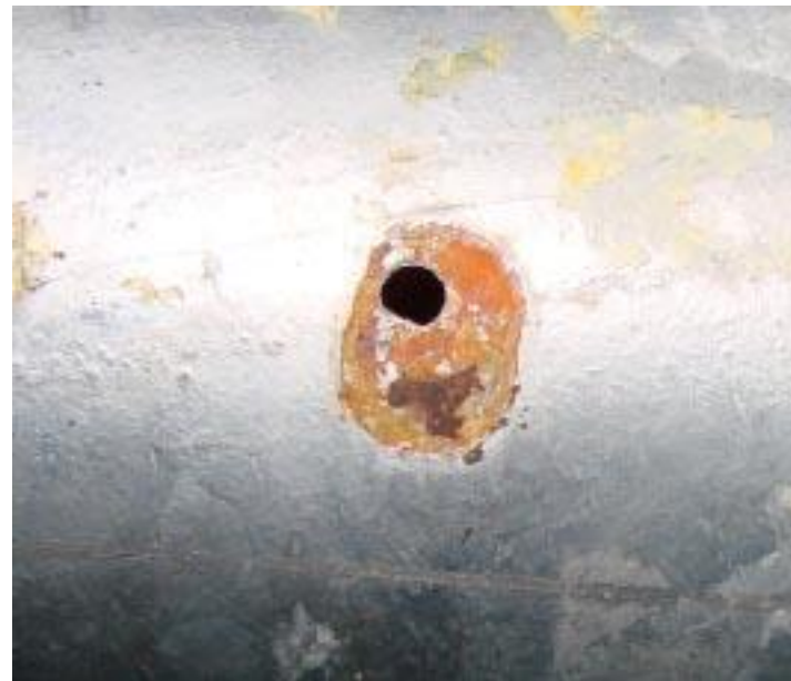
Galvanized Schedule 10 after only 18 months
