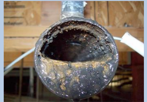
Dry sprinkler system, 5 years old
