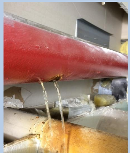
Dry sprinkler system with pinhole leaks.
